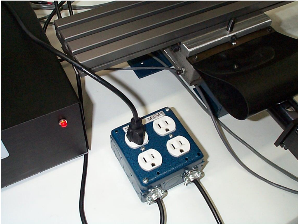
Fig. 3D – The Spindle and Auxiliary Relay Control Module.
